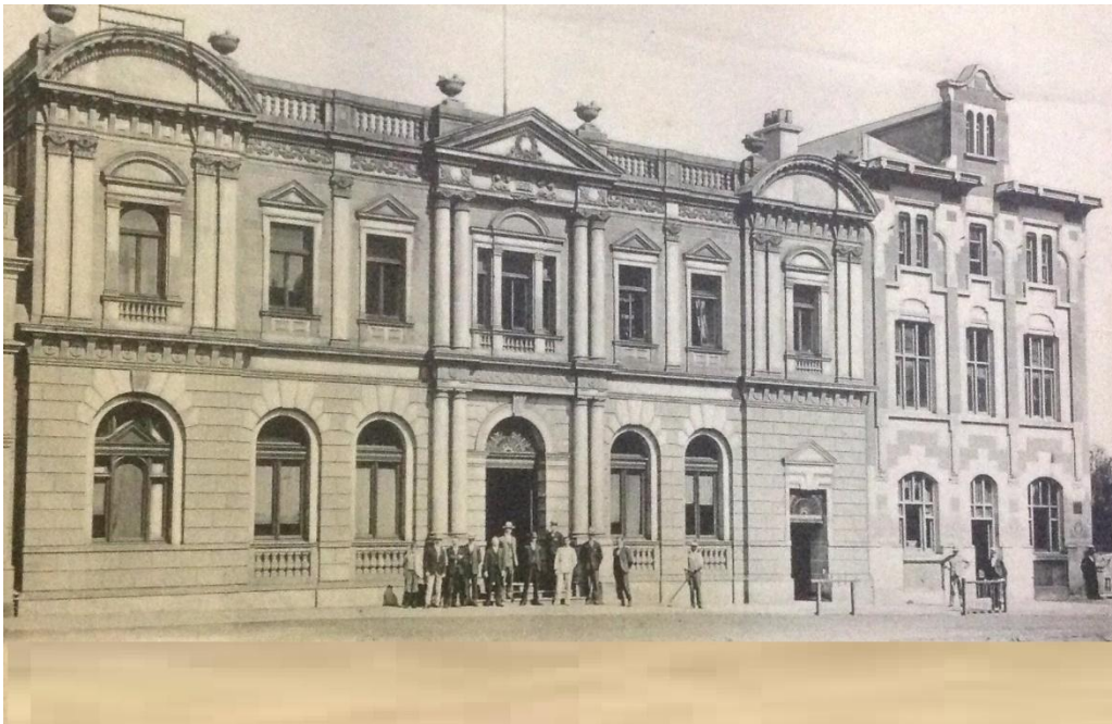
National Bank of the South African Republic, Pretoria. Source: The Heritage Portal
